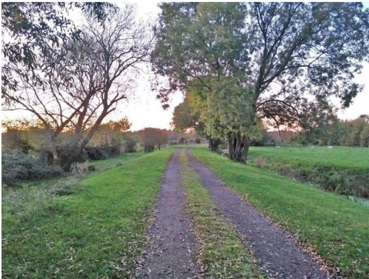
Figure 2: Much of the former rail alignment remains as an elevated embankment suitable for reinstatement (Photo: C. Ross 2019).
